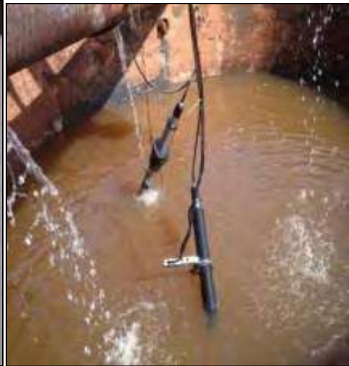
ETP Outlet flow meter
