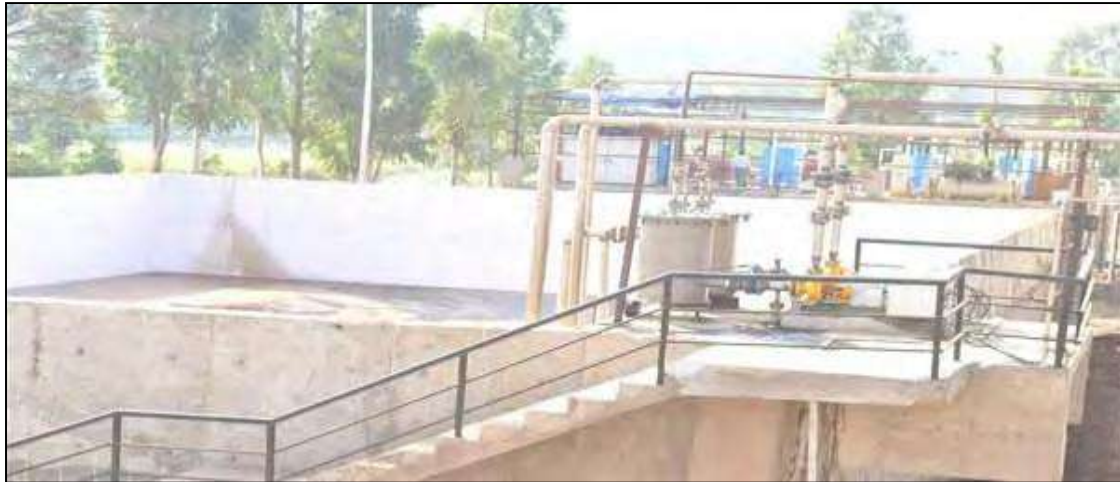
Five days Spent wash storage tank at Distillery
