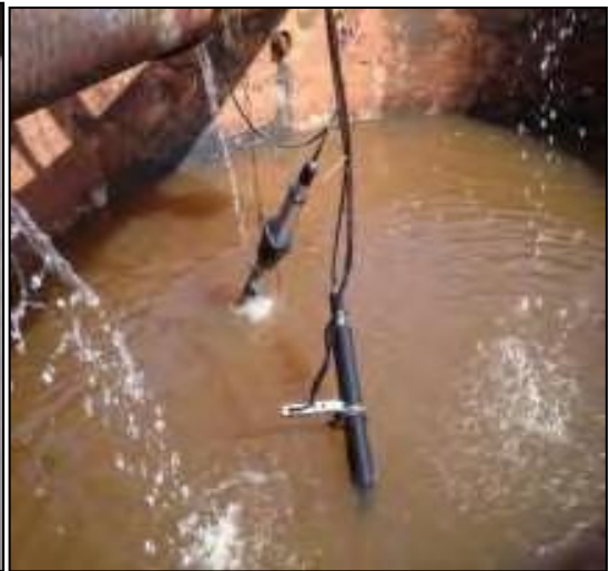
ETP Outlet flow meter
